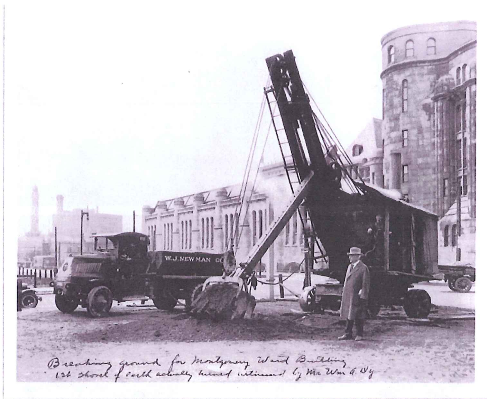
Montgomery Ward Memorial Ground-breaking 1925
