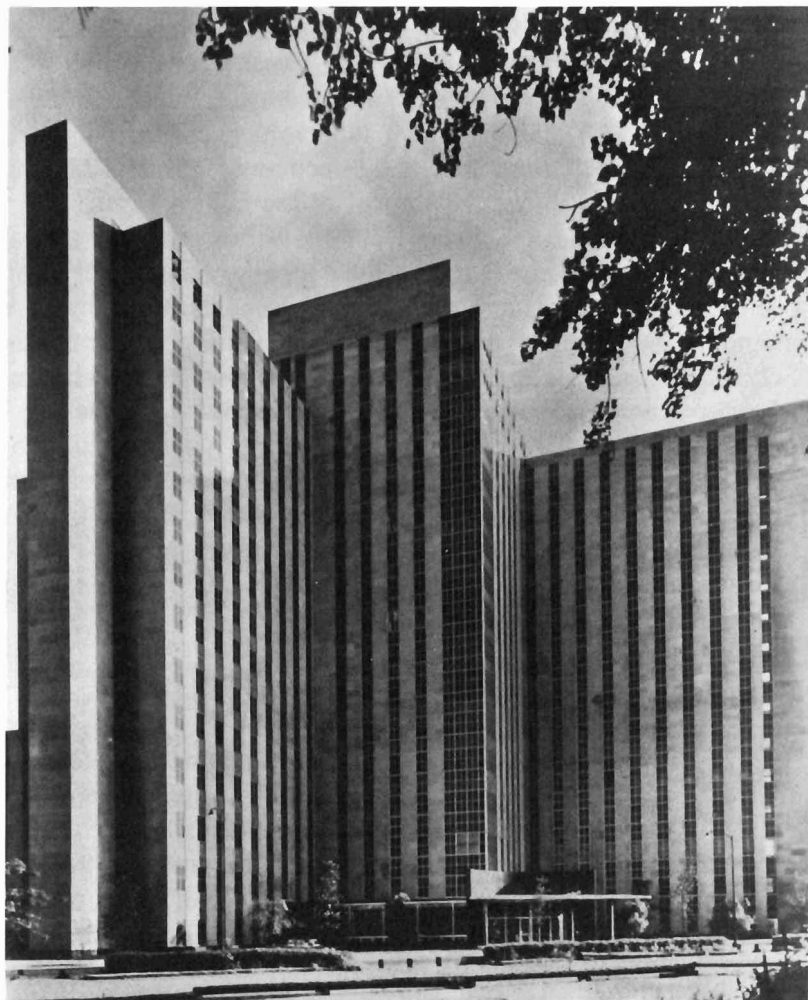
Veterans Administration Lakeside Hospital; erected 1954.
