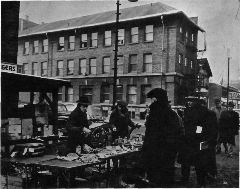
Chicago Maternity Center; erected 1904.
