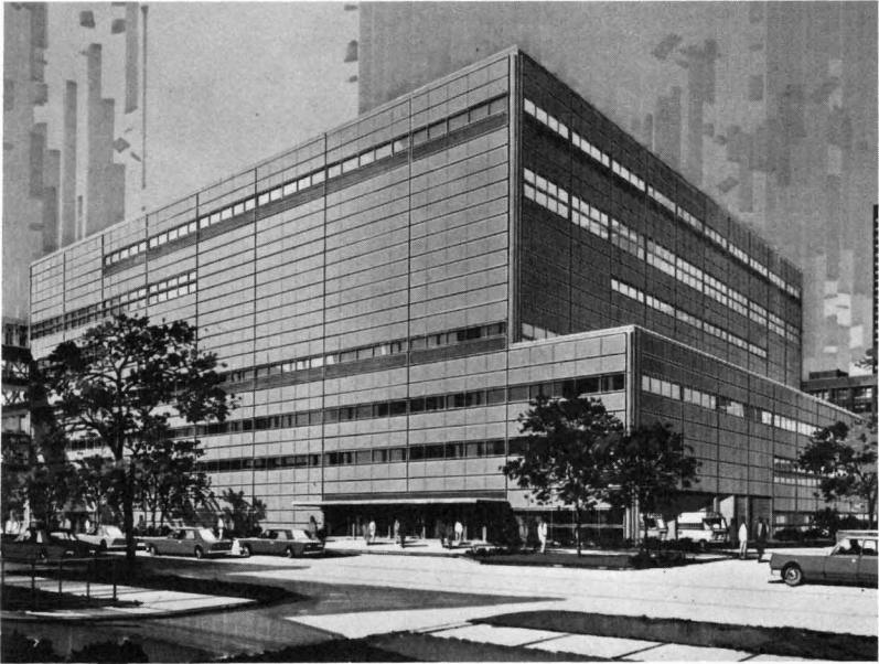
Health Sciences Building; erected 1979.
